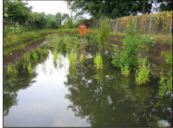
The wetland at Bruns Avenue Elementary in Charlotte treats stormwater runoff from the school and surrounding neighborhoods and provides an attractive landscape amenity.
