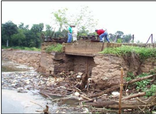
**Photo 1: Lake Conestee Dam, ca. 1892, on the Reedy River, Greenville County. View of dam from upstream with partially open gate, August 2000. Note dilapidated gate assembly and accumulated trash and debris.**
