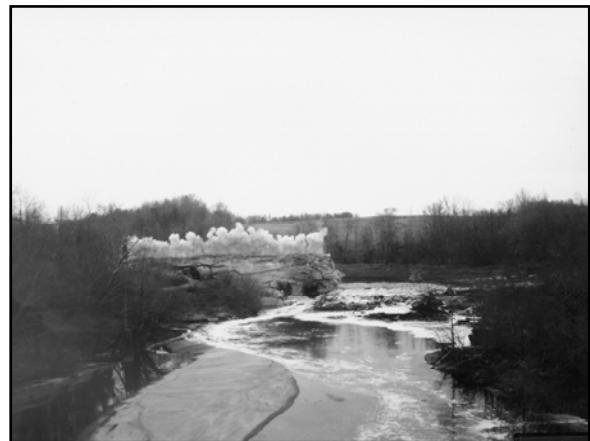
Photo 6: Tumblin' Shoals Dam Demolition, Dec 1970.
