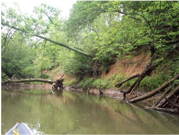
Photo 8: Effects from Erratic Hydroelectric Releases from Boyd Mill Pond Dam. On the Reedy River in Laurens County.
