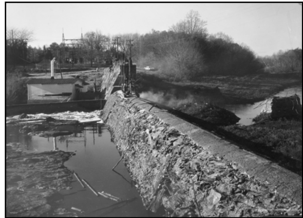
Photo 5: Tumblin' Shoals Dam Demolition, drilling for placement of explosives, Dec 1970.
